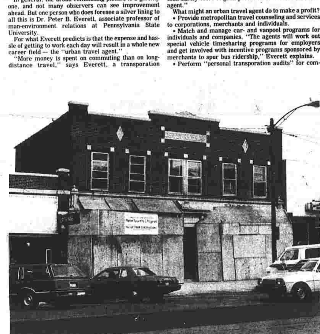
The Dewey Richman Building on Main Street (left) is blocked off from public view by the construction barricade in front of it, but there is a great deal of activity behind the barricade as the building undergoes conversion to offices that will be used by law firm of Phelon, Squatrito, and Fitzgerald. When the work is done the rear of the building, which abuts the Birch Street parking lot, will look like the sketch at right. A sunken atrium, with a ramp for use by handicapped persons, will lead into offices on the ground level. At the front, on the main level, the original center entrance will be preserved. Two recessed entrances will be built at either end as well.
